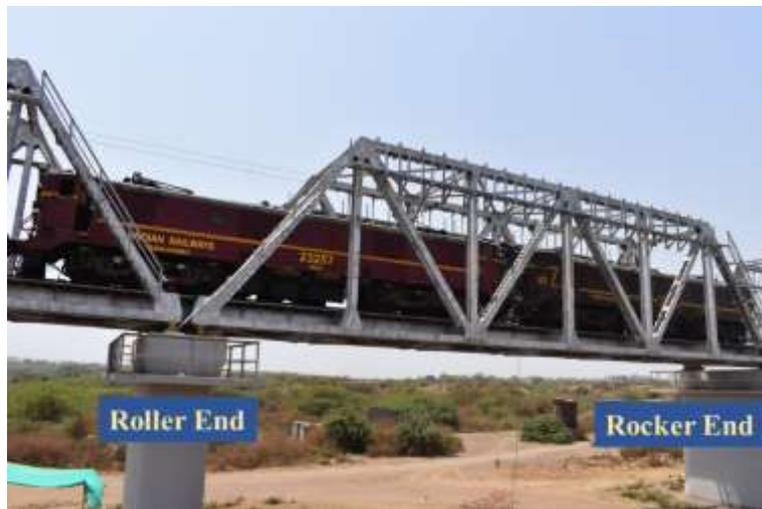
Fig. 13 Dual loco placed for maximum bending moment case
