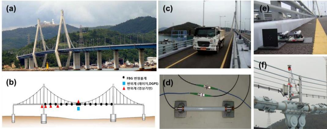
Fig. 17 Benchmark test on Sorok Bridge
