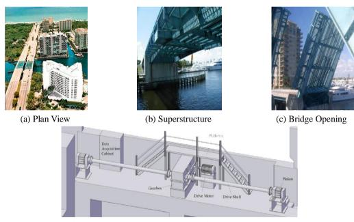
(d) Some of the Mechanical/Electrical System of Representative Movable Bridge
