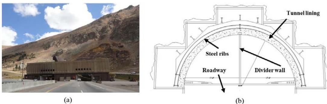
Fig. 2 Eisenhower Memorial Tunnel: (a) view of entrance and (b) view of the plenum
