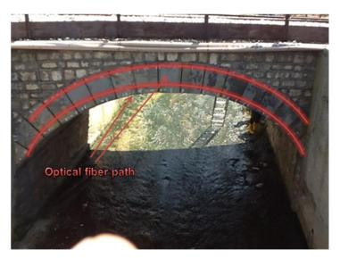
Fig. 6 Instrumented rail bridge (picture of "sea side"). The red curves indicate the path of the glued optical fiber
