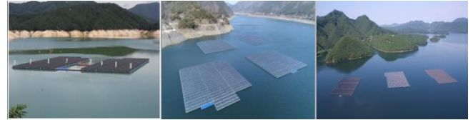
Fig. 1 Floating solar PV facilities of K-water (Kim 2018)
