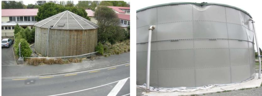
Fig. 1 Foundation sliding (right) and wall damaged due to sloshing motion (left) in Darfield earthquake (2010) (Courtesy of Timbertanks)
