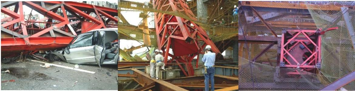
Fig. 1 Scenes of the tower-crane accident in the Taipei 101 Building caused by the earthquake
