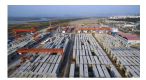
Fig. 16 Segment storage yard for the Leqing Bay Bridge
