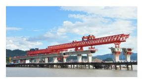
Fig. 14 Cantilever erection of the Leqing Bay Bridge
