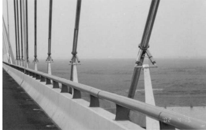
Fig. 13 Final installation of MR damper system
