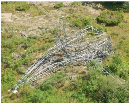
Fig. 1 Guyed tower failure (Hydro One report, 2006)
