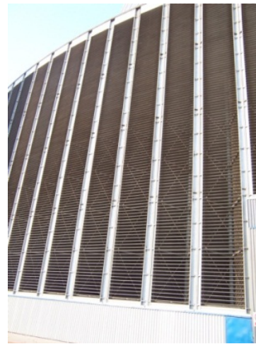
(b) Local structure of radiator shutters
