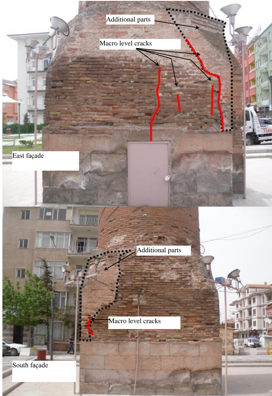
Fig. 6 Some damages on boot segment of Crooked Minaret
