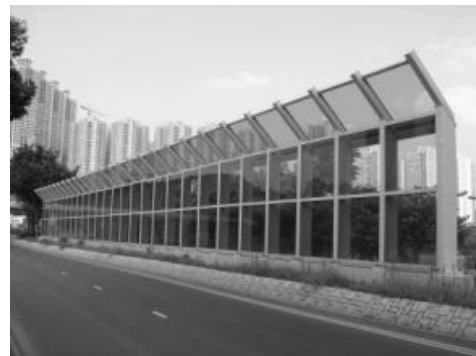
Vertical NMS with an inclined part at-grade (after Shum et al. 2011)
