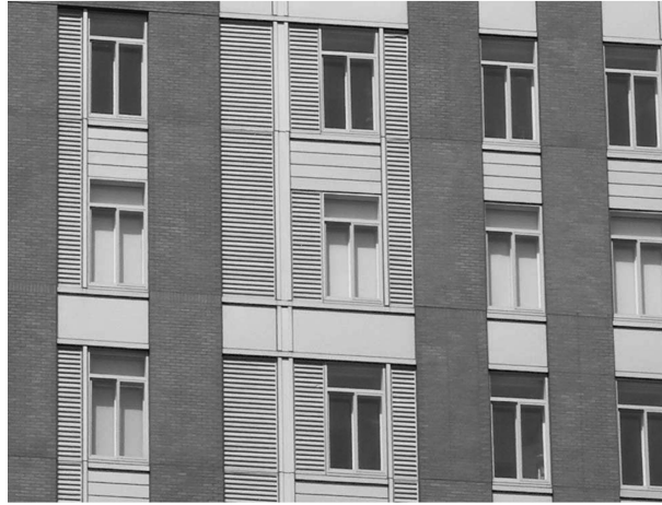
Fig. 1 A building wall with built in louvered panels
