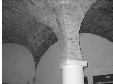
Fig. 3 A typical cross vaulted roof
