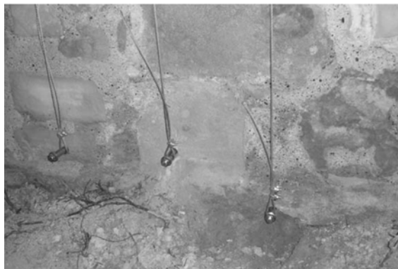
Fig. 11 Bolts used to fix the assembly at the bottom of the pier
