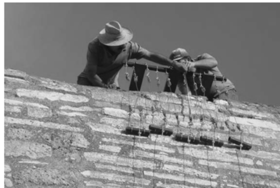
Fig. 9 SMA wires supported at the rigid base at the top of the pier of the aqueduct
