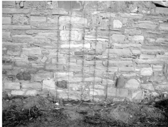
Fig. 10 Prestressing devices used to apply tension in the assembly
