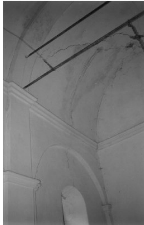
Fig. 6 Past intervention using steel bars
