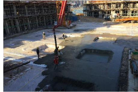
(c) Concrete pouring work image
