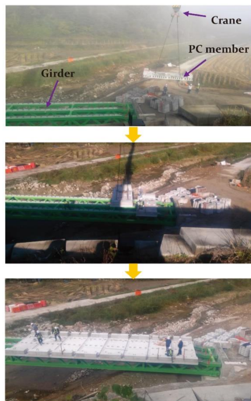
Fig. 20 Assembly process of PC members
