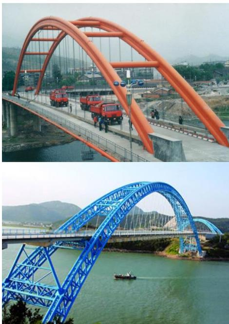
Fig. 1 Photos of CFST arch bridges
