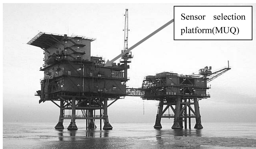
Fig. 9 View of JZ202-MUQ offshore platform
