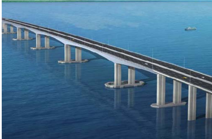
Fig. 8 The investigated continuous steel bridge
