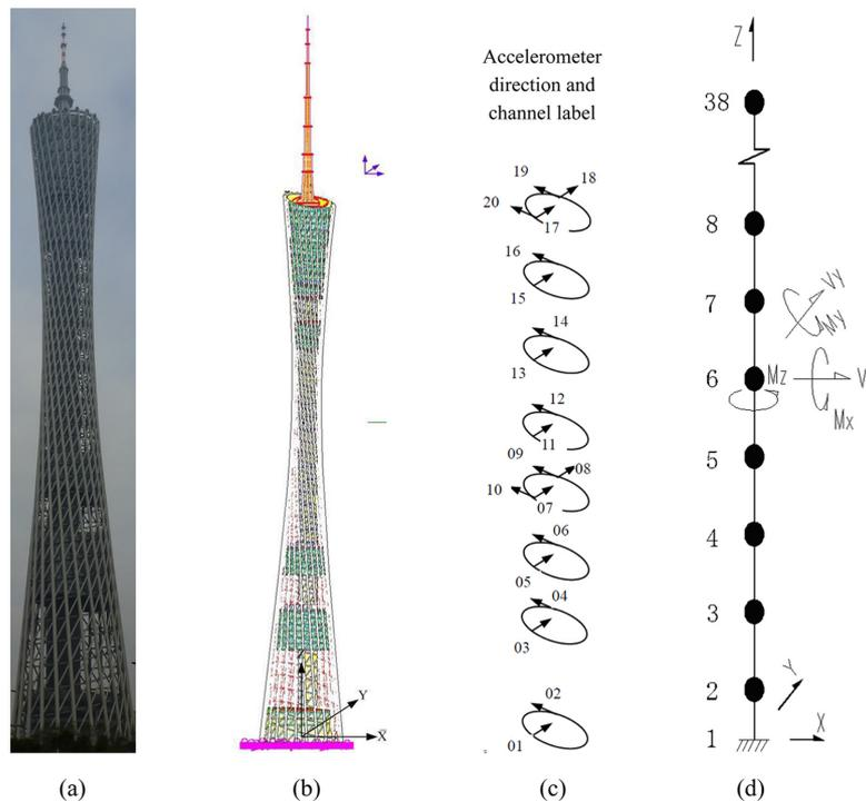
Fig. 1 The Canton Tower: (a) Actual structure, (b) full finite element model, (c) positions of installed accelerometers, and (d) reduced FE model (after Ni *et al.* 2012)
