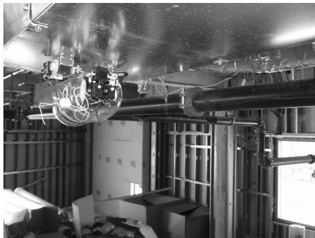
Fig. 8 MagGIE traversing galvanized ductwork
