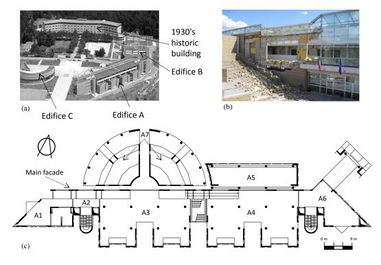
Fig. 5 Engineering Faculty of the University of L'Aquila: (a) overview of the buildings' set, (b) photo of the main facade of the Edifice A damaged during the L'Aquila Earthquake and (c) plan map of Edifice A
