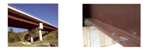
Fig. 15 Composite road bridge monitoring by a portable prototype BOTDA system
