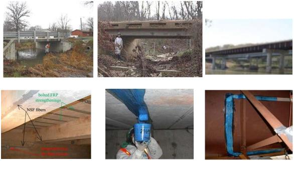
Phelps Country bridgeWalters Street bridgeBridge A6358Fig. 13 Short-span bridges monitored by BOTDR technique based on AQ8603 system
