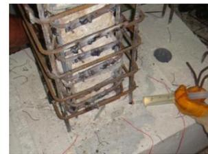
(c) insertion of epoxy resin
