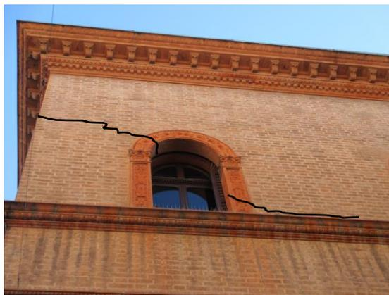
Fig. 4 Diagonal cracks on external windows
