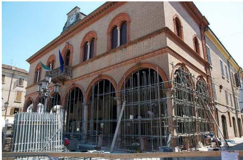
Fig. 13 Scaffolding in the North-West side of the Facade during May 29<sup>th</sup> Shock
