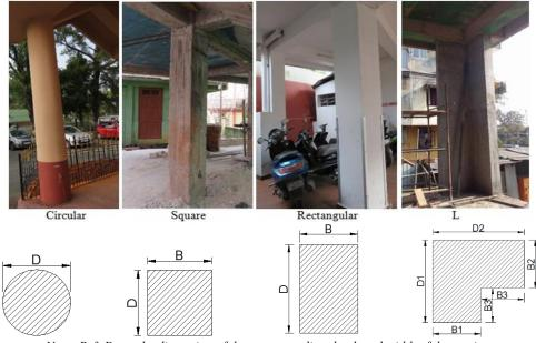
Note: B & D are the dimension of the corresponding depth and width of the sections
