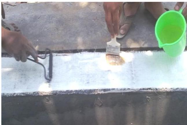
Fig. 5 GFRP lamination in progress
