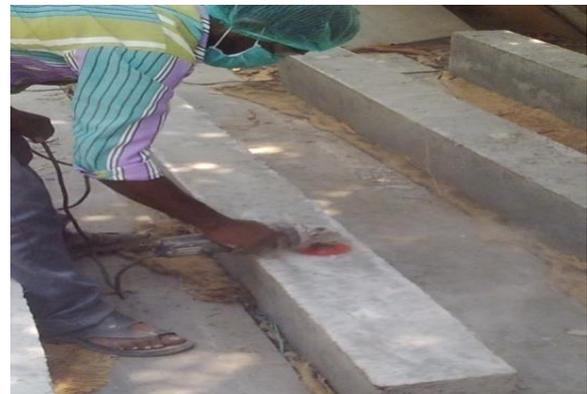
Fig. 4 Surface grinding in progress
