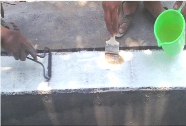
Fig. 5 GFRP lamination in progress
