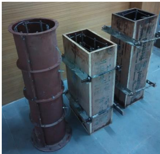
Fig. 3 Formwork for circular, rectangular and square column
