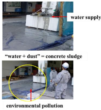
Fig. 1 Problem of water-cooled concrete cutting method
