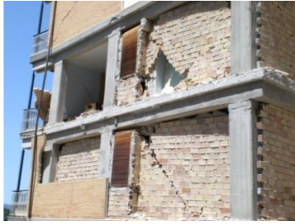
Fig. 1 Failure of infills due to poor infill-frame connection, L'Aquila, Italy, earthquake of 2009
