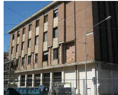
Fig. 4 Failure of the external layer of the infill, Emilia, Italy, earthquake of 2012
