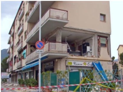
Fig. 2 Failure of infills at the first storey, L'Aquila, Italy, earthquake of 2009
