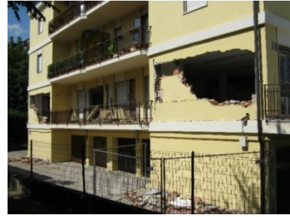
Fig. 3 Expulsion of the infill at the first storey, Emilia, Italy, earthquake of 2012
