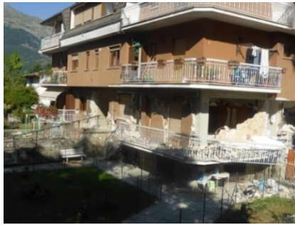
Fig. 5 Infill failures at the first storey, Central Italy earthquake of 2016
