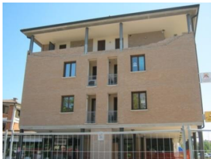
Fig. 6 Failure of the parapet at the top storey, Emilia, Italy, earthquake of 2012
