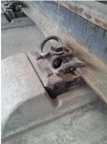
Fig. 1 Rail fastener system of slab track system
