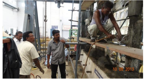
Fig. 3 Grouting done in retrofitted frame
