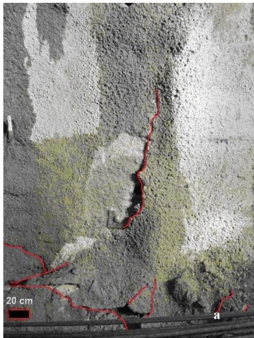
Fig. 8 The cracks of the shotcrete due to the high deformation
