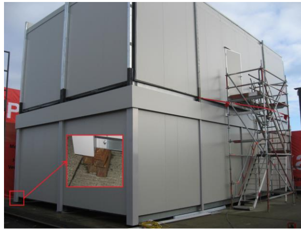
Fig. 1 External view of the two-module prototype test building
