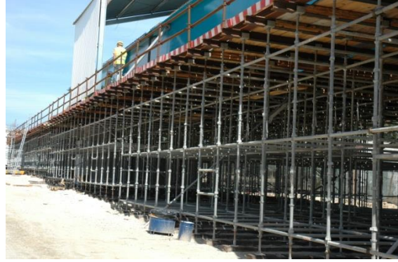
Fig. 6 Example of bridge falsework Cuplok® systems
