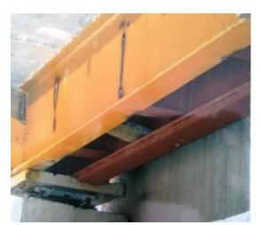
Fig. 11 Remedial Measure-I Implemented in real (i.e., as buit) pipe-rack
