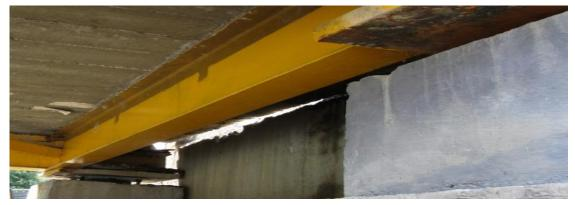
Fig. 3 Eccentric placement of cross girder over the bearing plate
