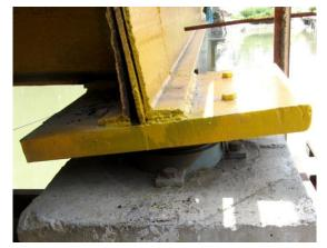
Fig. 2 A visible tilt in the bearing plate
