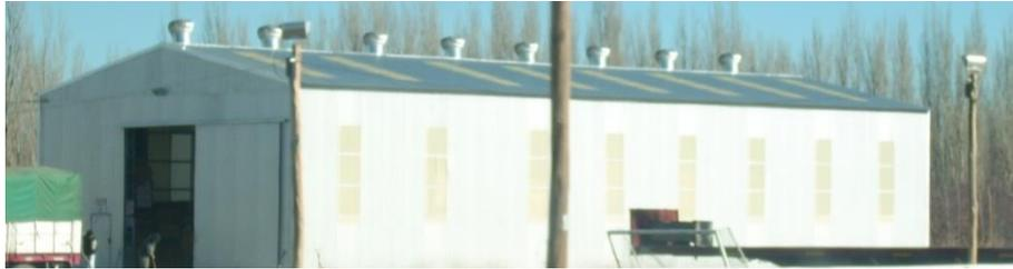
Fig. 3 Gable roof storehouse with sinusoidal plate cladding
