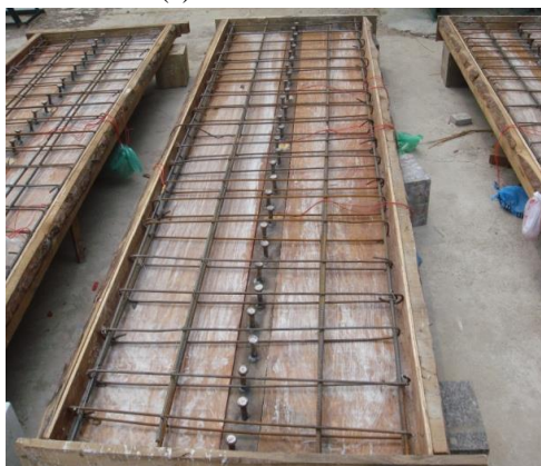
(c) Formwork for concrete slab
