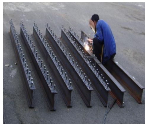
(b) Welded joints
