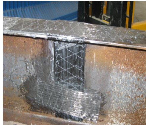
(f) Paste CFRP sheet and U-shaped hoop
