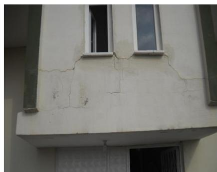
Fig. 13 Damage arose from heavy cantilever in the reinforced concrete building
