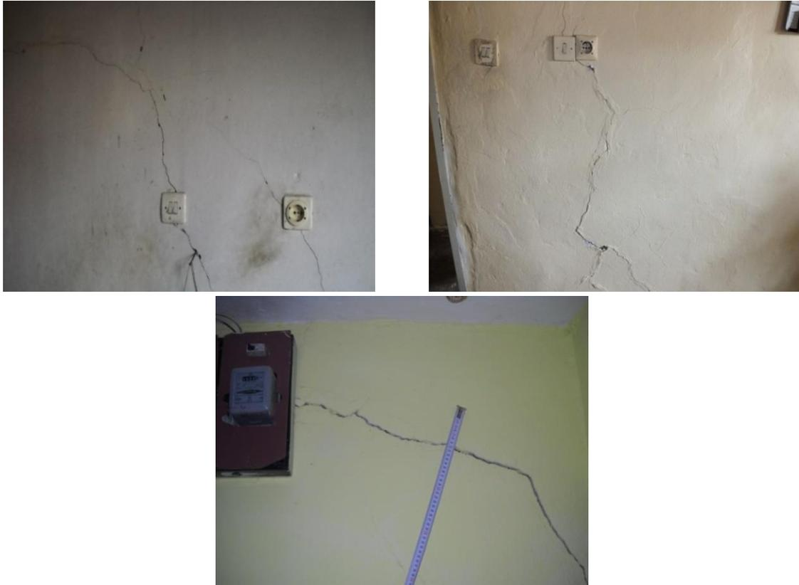
Fig. 10 Diagonal and vertical cracks arising from deficiencies electrical wirings
