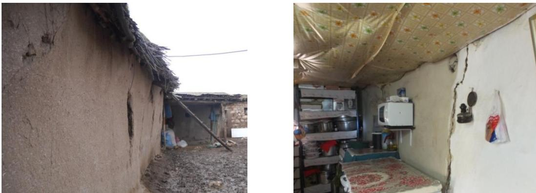
Fig. 5 Out of plane mechanism arose from blast-induced vibration for various adobe buildings
