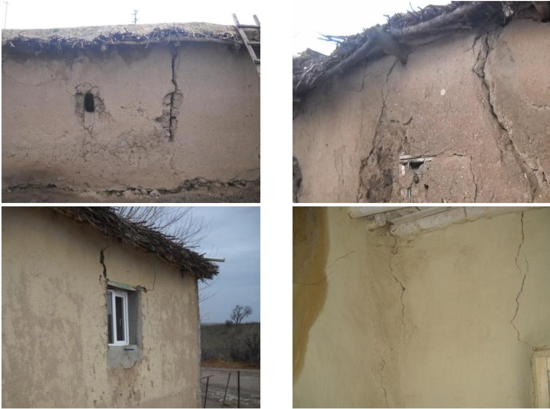
Fig. 3 Flexural failure and diagonal crack at various adobe buildings
