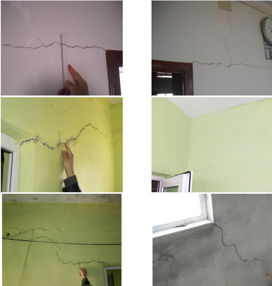
Fig. 14 In plane failures in various reinforced concrete buildings
