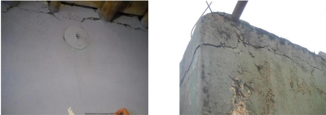
Fig. 7 Sliding failures in different brick masonry buildings
