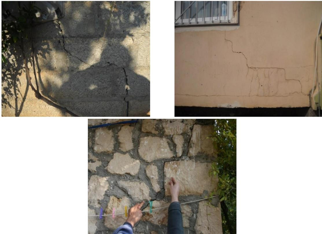
Fig. 8 Diagonal stepped cracks in various brick and stone masonry buildings
