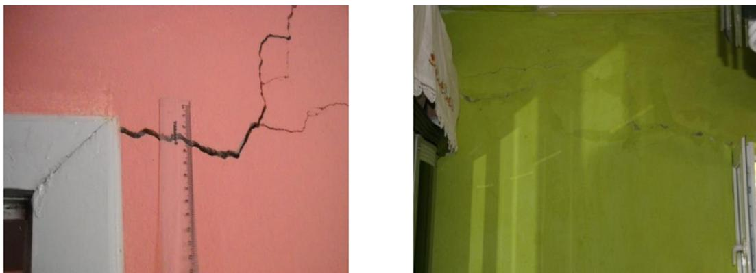
Fig. 9 Diagonal shear cracks in different brick and stone masonry buildings
