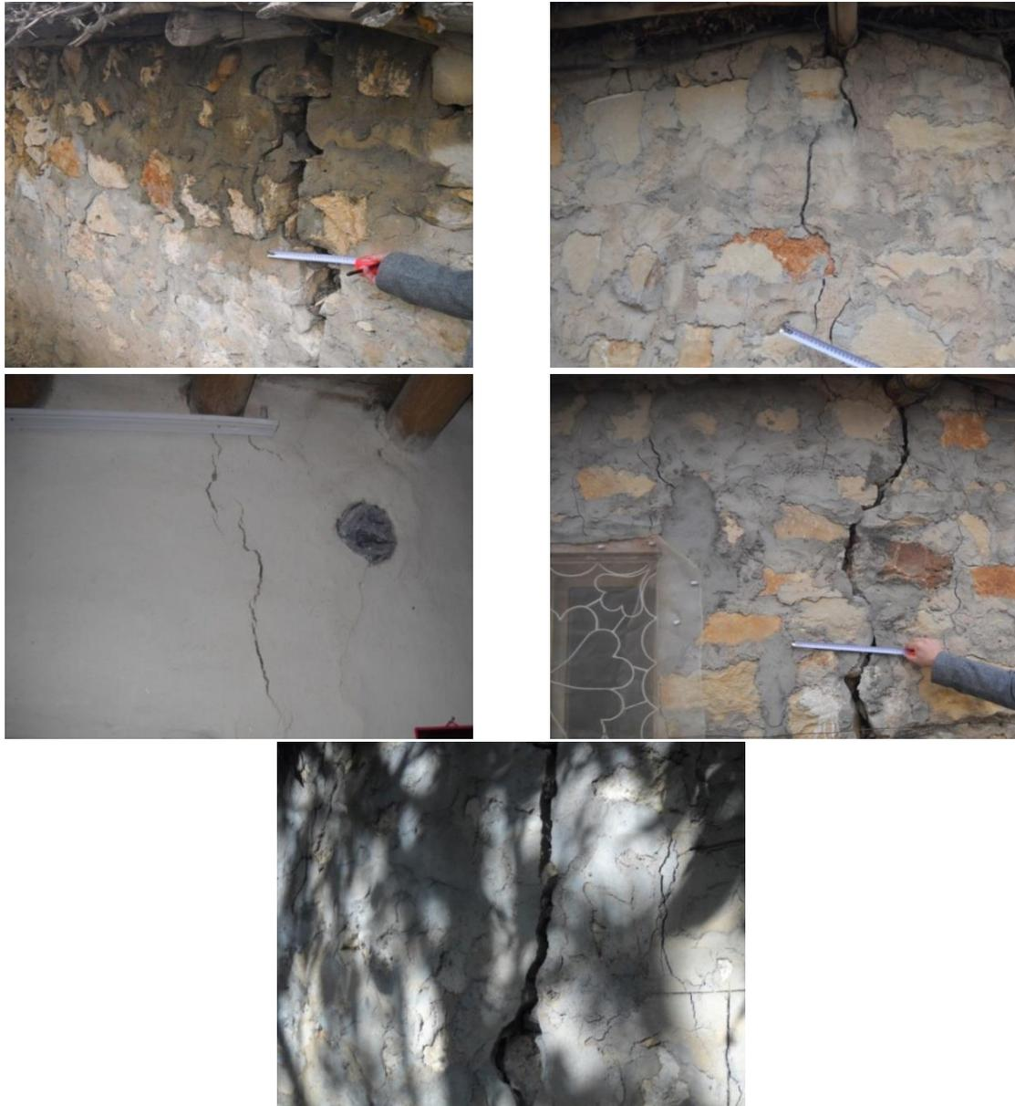
Fig. 11 Flexural cracks in various masonry buildings
