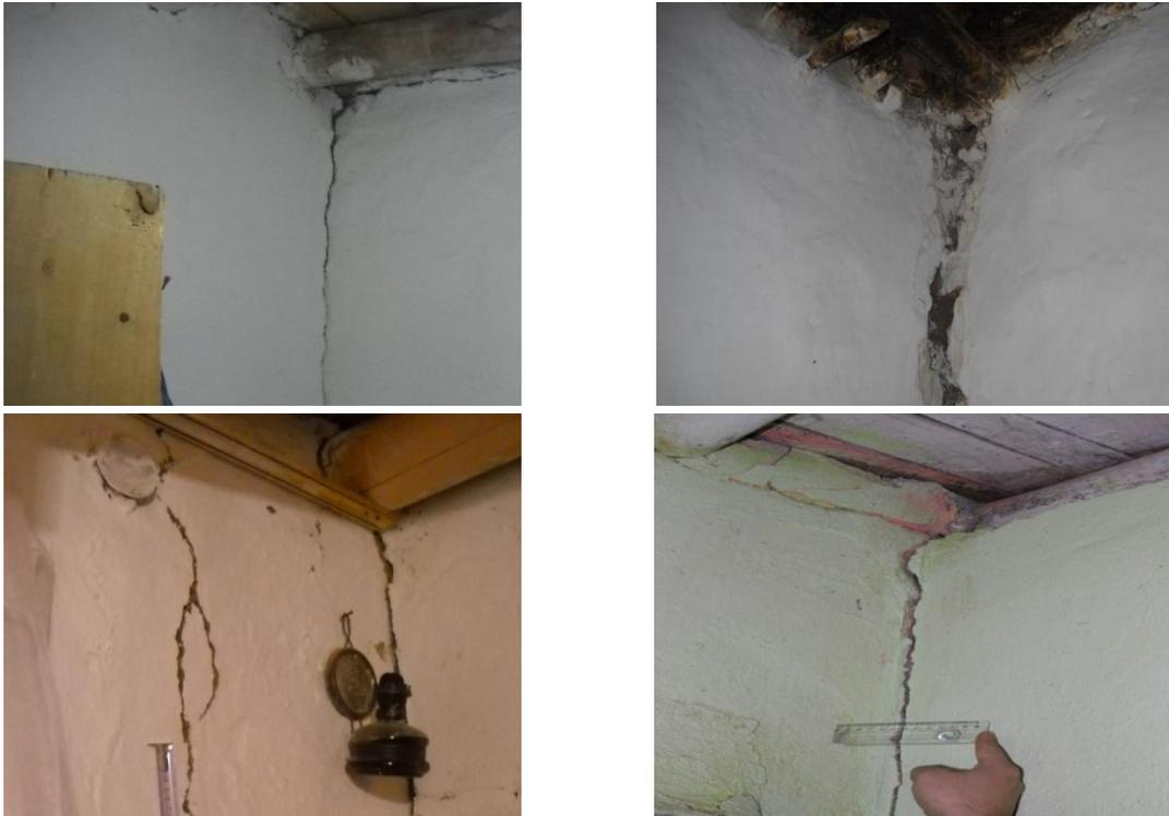
Fig. 4 Damages at corner walls of adobe buildings
