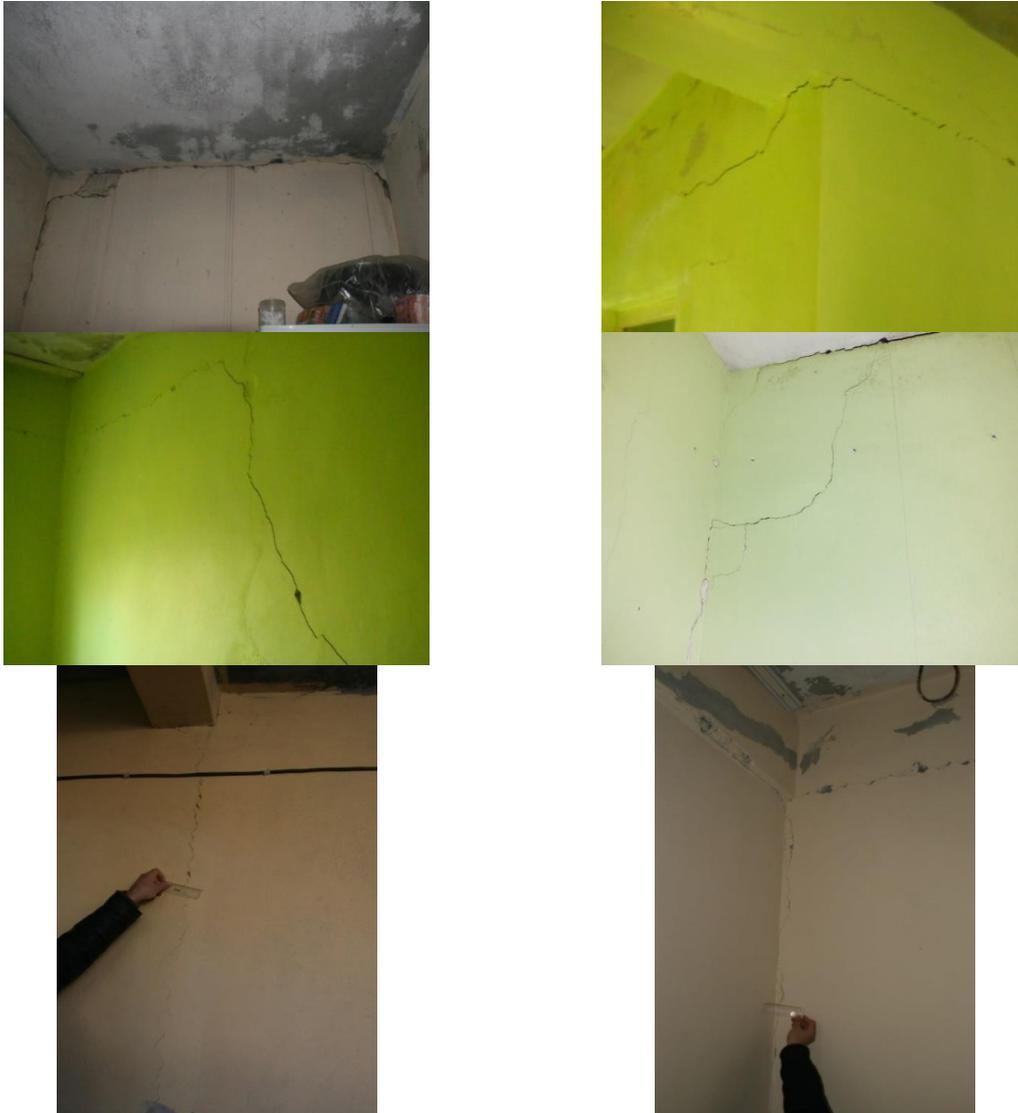
Fig. 12 Damages to infill walls in various reinforced concrete buildings
