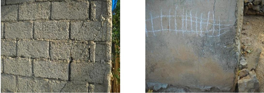
Fig. 6 Corner damages at various brick masonry building
