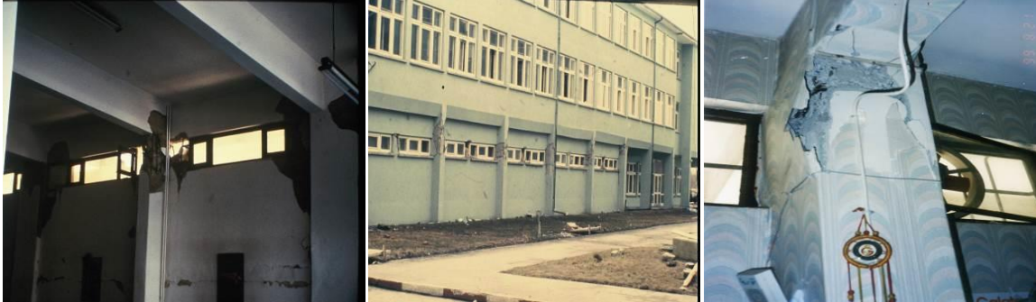
Fig. 1 Columns showing short column behavior and damage due to band windows
