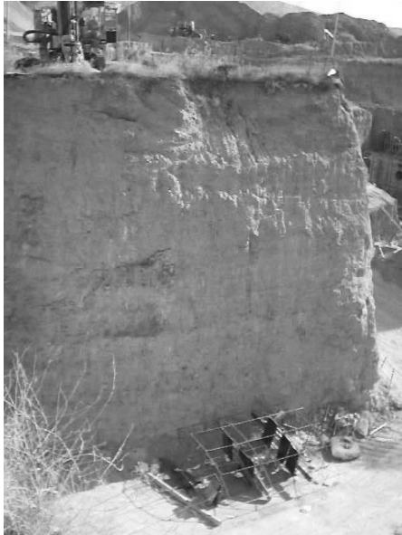
Fig. 7 Very cohesive conglomerate formation as Olympic Wrestling Hall foundation
