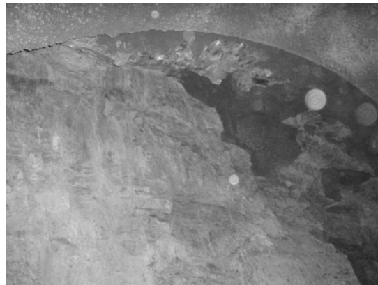
Fig. 6 Chloritic schist rock mass during tunneling of Symbol Mountain at Strymonas-Kavala's part of Egnatia Highway at Northern Greece
