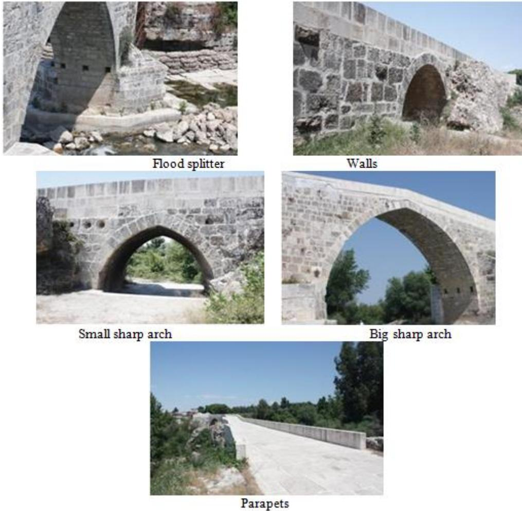
Fig. 7 The architectural members in Aspandos Masonry Arch Bridge
