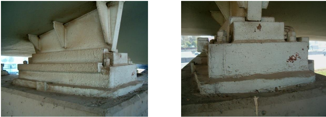
Fig. 4 Steel bearings of the superstructure
