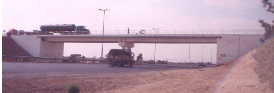
Fig. 2(a) Picture of concrete highway bridge comprised of two 23 m spans
