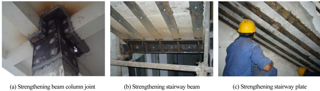
Fig. 8 Seismic repair of the damaged structural components
