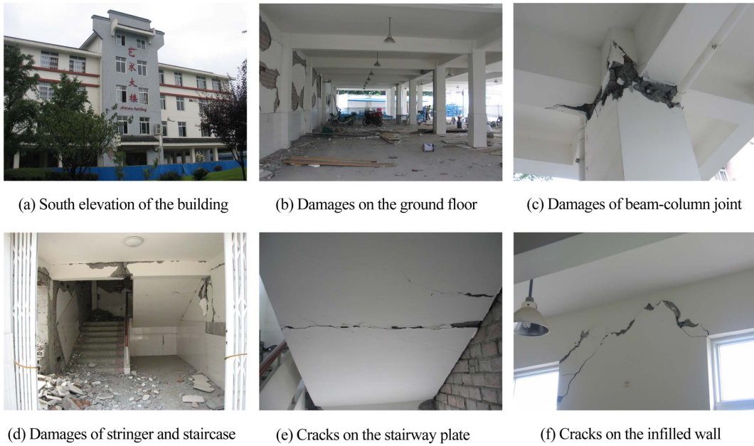
Fig. 7 Damages of a framed structure in the Wenchuan earthquake
