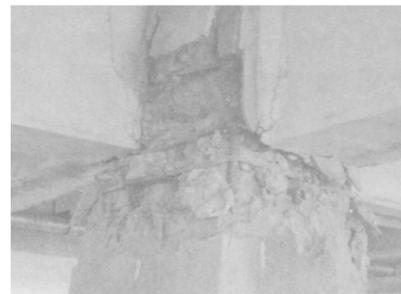
concrete cover spalled, joint core concrete seriously damaged, and column longitudinal rebars deformed
