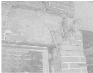
the serious diagonal damage of the joint was mainly due to the lack of joint transverse reinforcement
